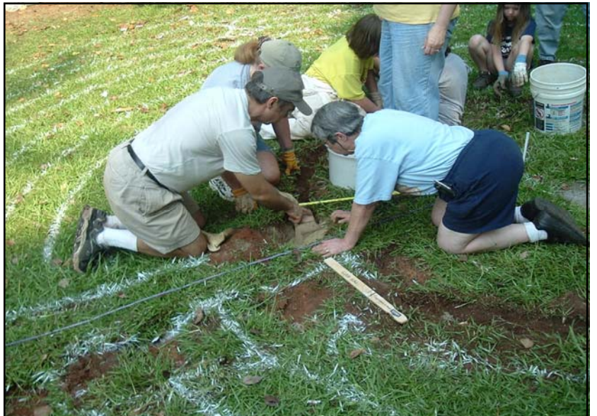
"Setting the cornerstone - the second most important task. From this point all other stones will be aligned."
